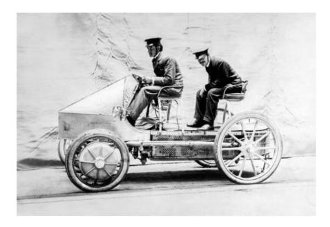
Ferdinand Porsche, the eponymous founder of the company, made the world's first hybrid electric vehicle...in 1899. The Lohner-Porsche "Semper Vivus" was essentially an electric car with an internal combustion motor used as a generator. It was also the first car with brakes on all four wheels. From Thrillist
